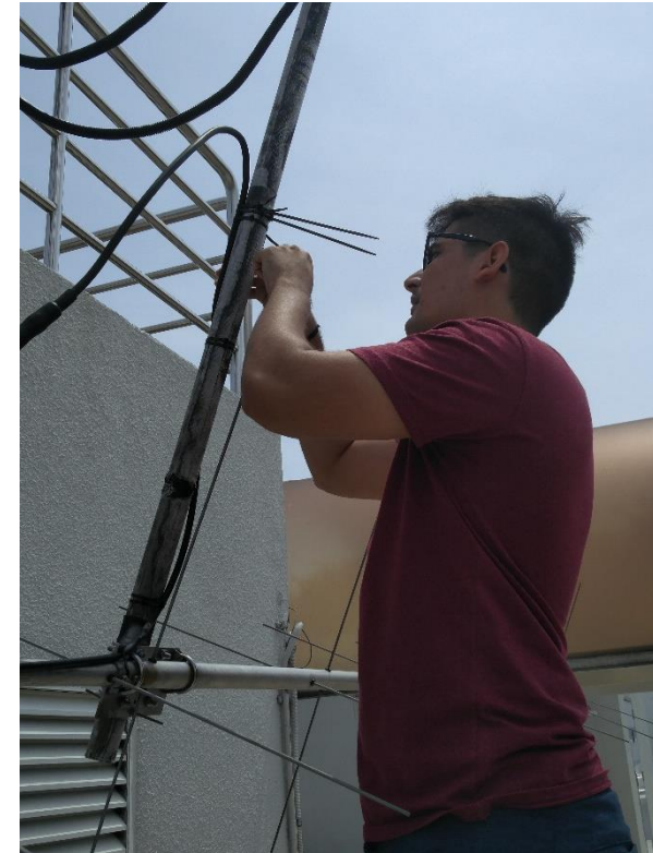
Ground Station: Cabling reworks.
