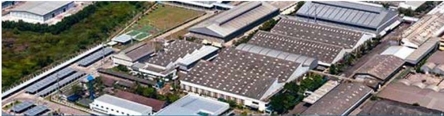
Industrial and Urban Infrastructure
